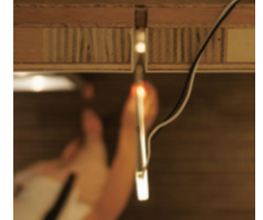
3/ Installation of the light appliance
